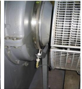
Spear valve conversion to hydraulic actuation
