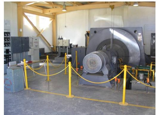
A view of the governing equipment in relation to the existing plant. The hydraulic module stands close to the turbine, and the governor panel is located at the end of the existing line of panels & switchgear
