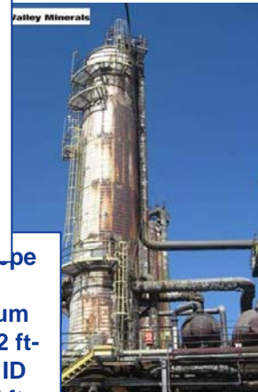
2008 Demonstration at SV Minerals - 50MW, includes new solvent (RS1), new packing material strategy, steam reduction
