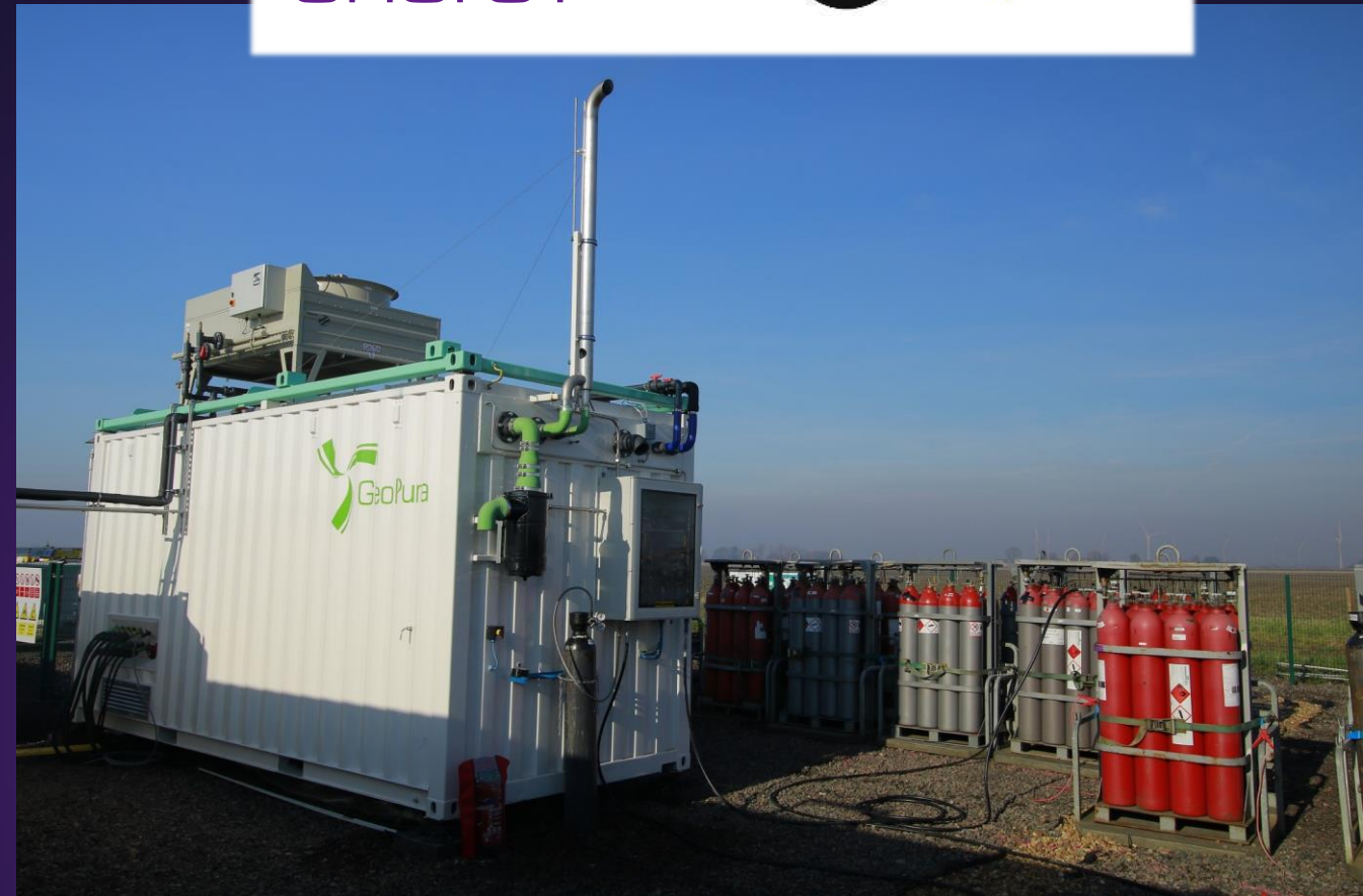
Photo: GeoPura Hydrogen Power Unit (HPU) at a customer site providing off-grid green electricity from green hydrogen via a PEM Fuel Cell system.
